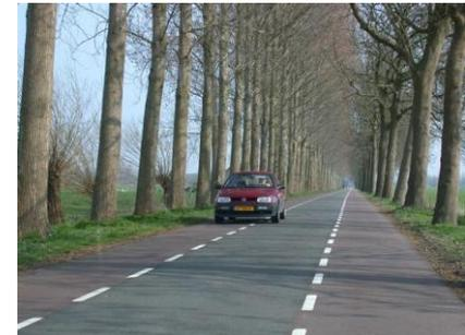
Wrong: no marking at roadside, no speed hump (road width >4,5m)
